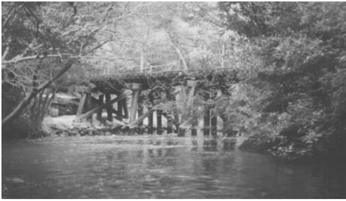
Railroad bridge over the Menantico Creek
